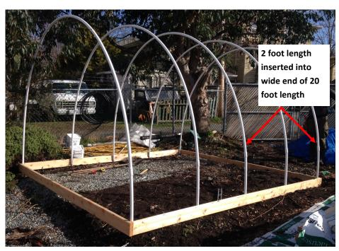
The two 20 ft long stabilizing side hoops were attached to the corners of the base with metal strapping, causing them to bend parallel to the side of the greenhouse.
